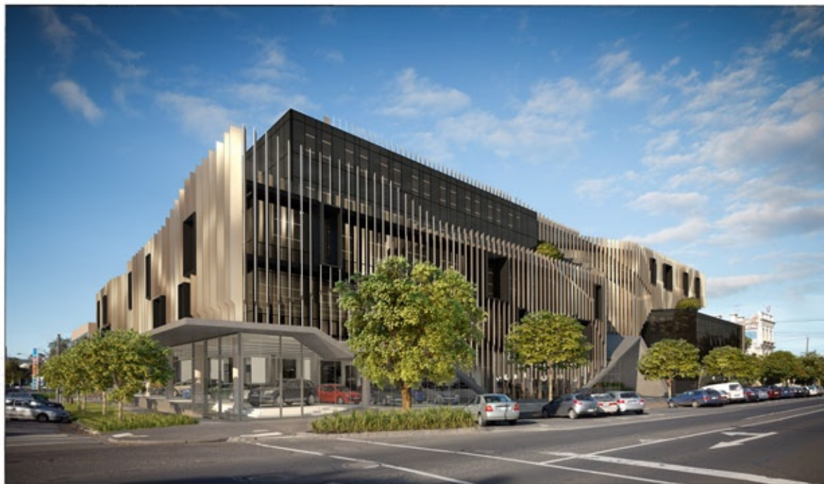
The Shearman family plans to build a retail and commercial development at 89 Moray Street in South Melbourne.
